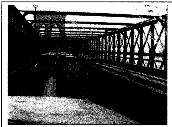
Photo 1: Road section sprayed by the FAST system
