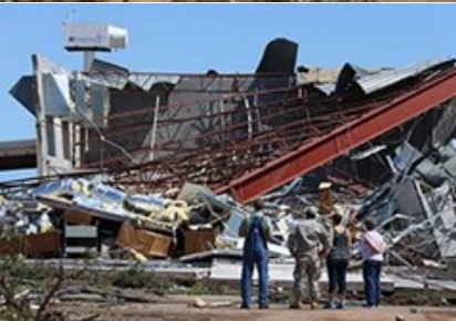
Recent Tornado Damage in Moore, OK
