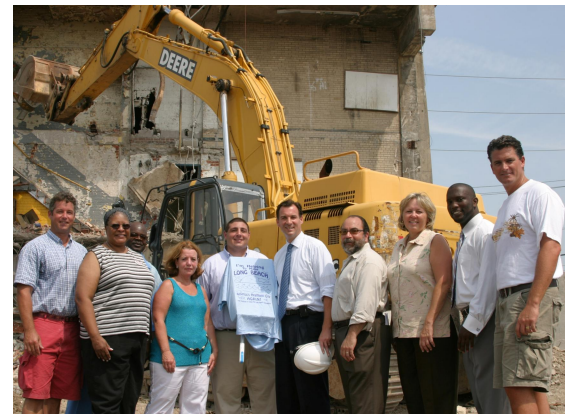
CE Suozzi with citizens of Long Beach at the incinerator demolition
