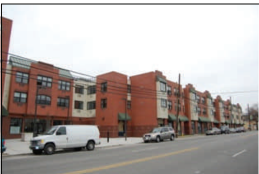
The Bluestone Organization developed Site A the "Gateway to New Cassel". This three-story building holds 57 rental units over commercial space
